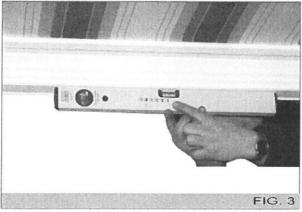
6 Using a level, check that the terminal is horizontal. If not, adjust the support screw for the arm that is not level using the procedure indicated above.
